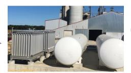
LNG Storage and Vaporization equipment to create Virtual Pipeline
