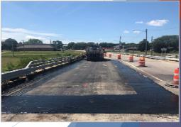
Wax-Modified Hot Applied Asphalt Tack Coat (WMT)
