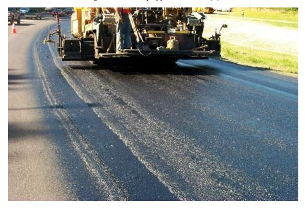
Figure 10. An appropriately applied tack coat [10]
