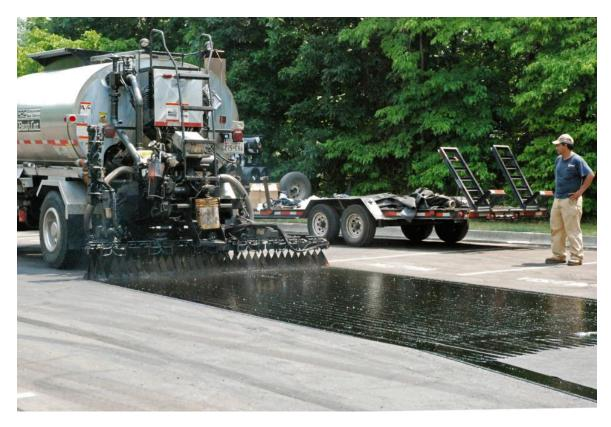
Figure 9. A heavily applied tack coat [9]
