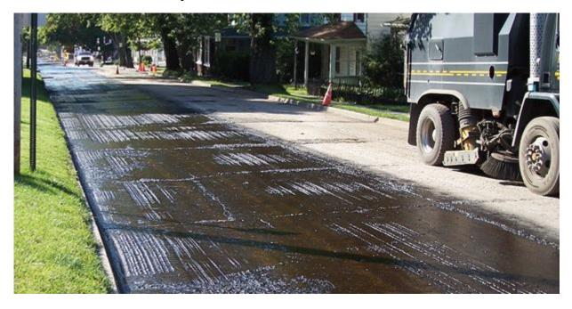
Figure 1. A tack coat applied to the first layer of pavement [1]
