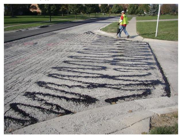
Figure 8. A lightly applied tack coat [8]
