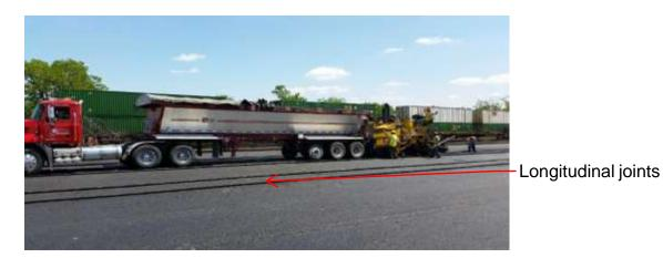
Figure 2. Asphalt paving operation with a paver and flow boy trailer.
