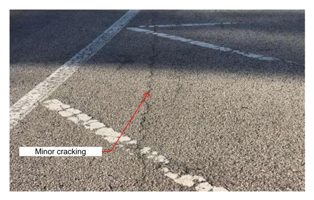
Figure 7. Minor longitudinal crack.
