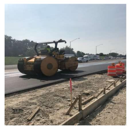
Figure 5. Rolling over asphalt concrete.
