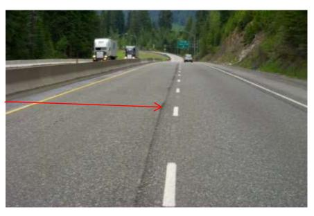
Crack formation at the longitudinal joint
