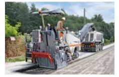
A top layer is milled off the existing pavement to provide a relatively smooth surface on which to pave. Milling is also commonly used to remove a distressed surface layer from an existing pavement. Milling machines are the primary method for removing old hot mix asphalt pavement surface material before the overlay. They can be fitted with automatic grade
