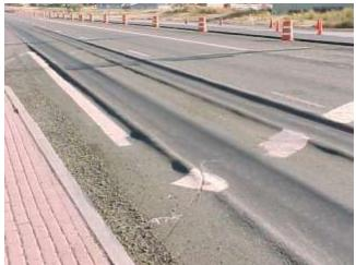
Figure 1: Pavement Rutting (Pavement Interactive n.d.)
