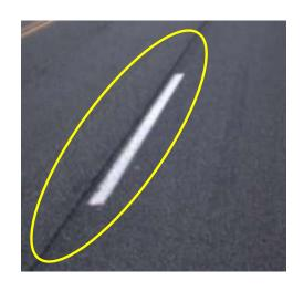
Minor longitudinal joint cracking & separation
